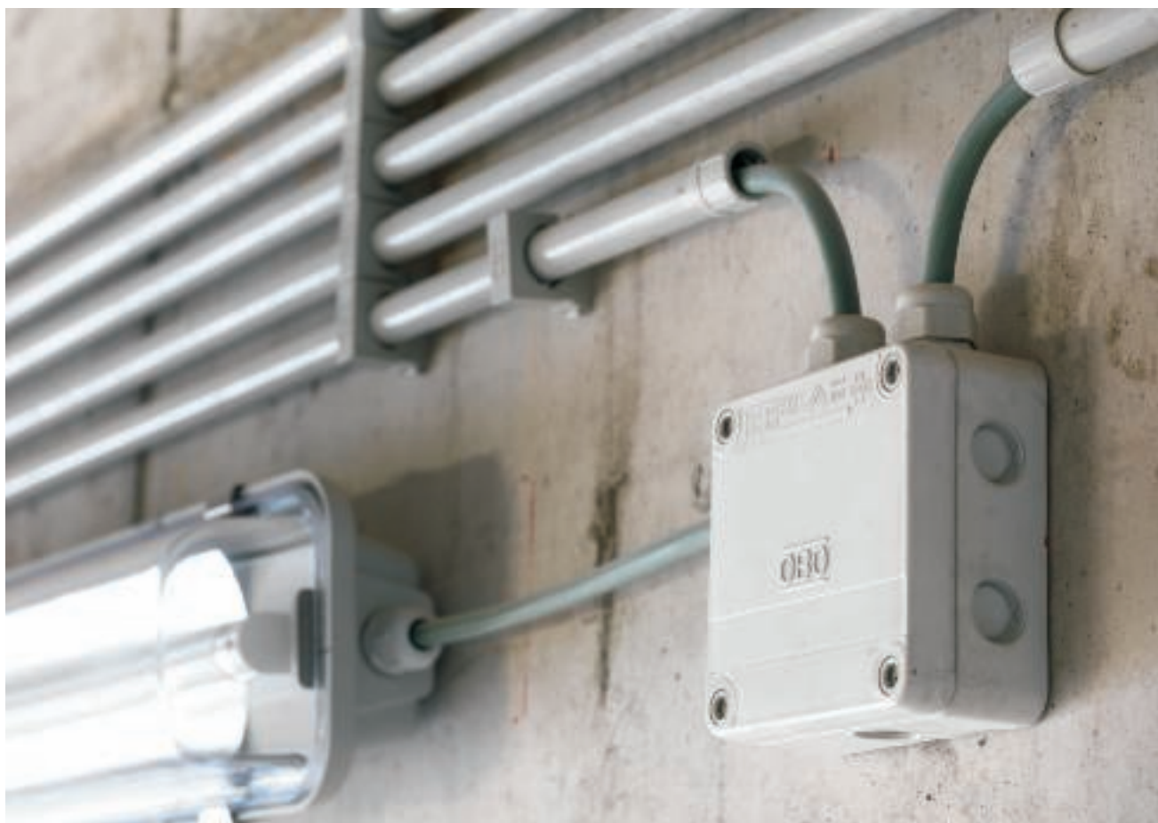
Aquasit - cold casting compound for junction boxes, protection rating IP68
